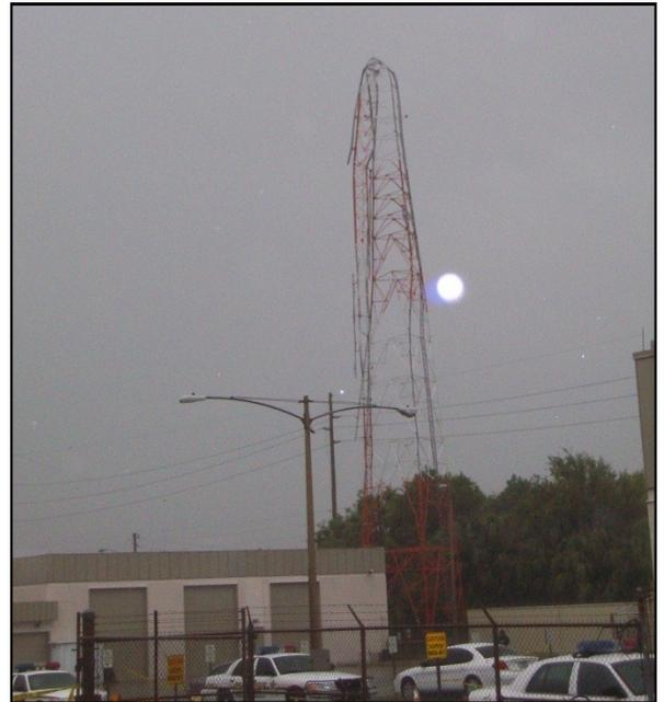
Tower collapse at Position 3. Winds near the ground estimated at 60 MPH while winds at top of tower estimated at over 110 MPH.
